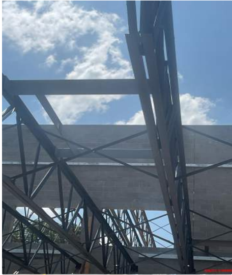
Relief Angle installed and RTU support set
