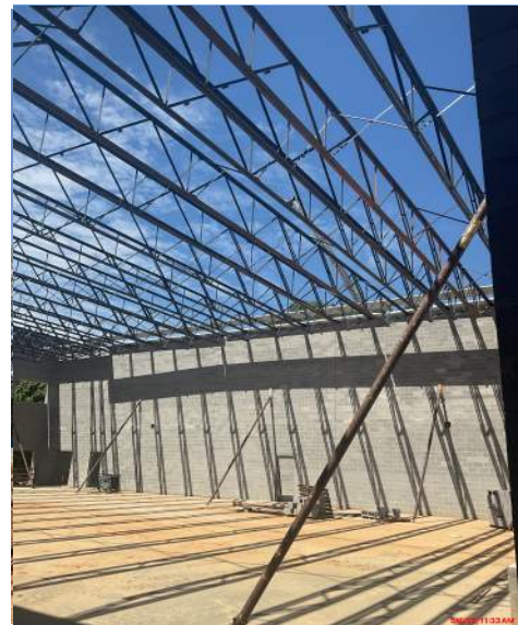
Steel joists installed
