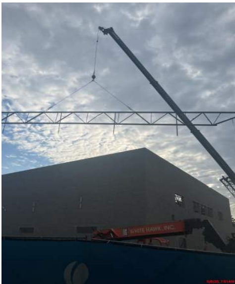
Crane setting steel joists in place
